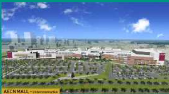
AEDON MALL - under construction
